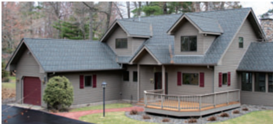
■ The profiles of the Vintage Slate Shingle (above) and Granite Shake (right) provide a heavy, multi-dimensional appearance at only 125 and 150 pounds per square, respectively.
