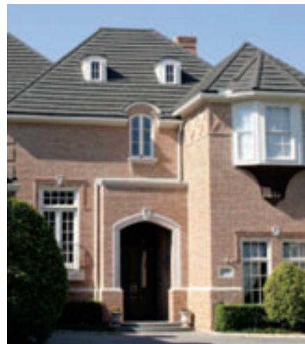
■ The profiles of the Vintage Slate Shingle (above) and Granite Shake (right) provide a heavy, multi-dimensional appearance at only 125 and 150 pounds per square, respectively.
